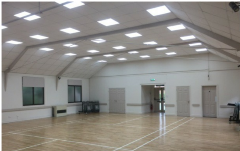
The newly renovated Church Hall
